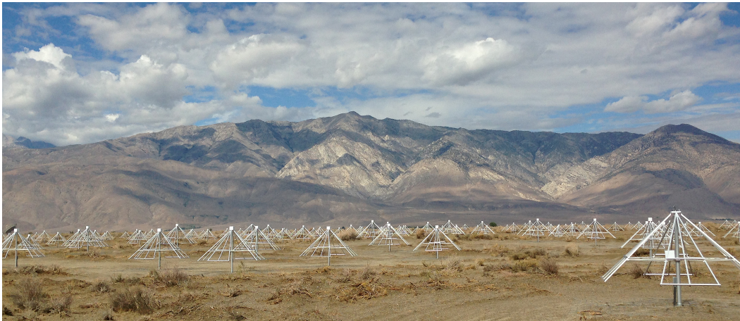
Figure 2.1: A photograph of the OVRO-LWA, taken from within the 251-element core, facing east towards the White Mountains. On the west side of the array is the Sierra Nevadas. The radio observatory's placement within the Owens Valley, shielded on either side by two large mountain ranges, creates a comparatively clean RFI environment. The predominant sources of RFI are the FM band above 88 MHz, short wave reflecting off the ionosphere below 25 MHz, and RFI associated with power-lines running along the valley that is broad-band in nature.
